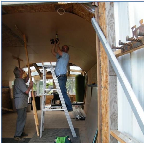
Dan Ellis & Martin installing curved hardboard ceiling panels which will be painted blue with white clouds.
